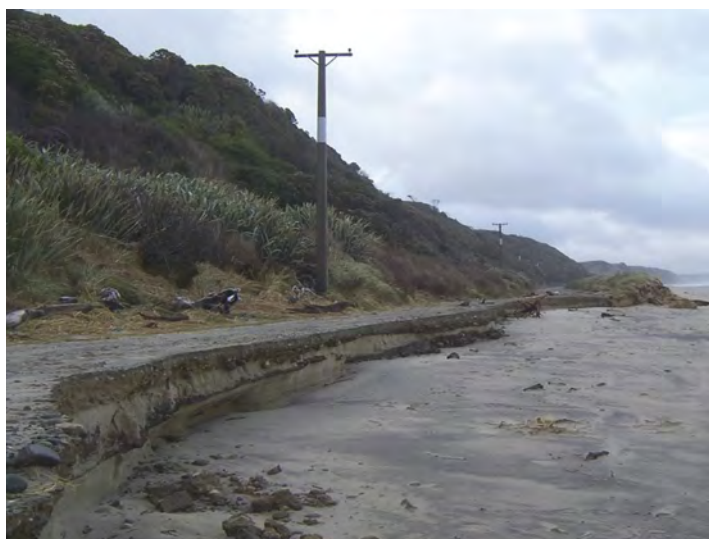
Sections of the Papatotara Coast Road, which were badly damaged by storms. Council is to reposition the road.
